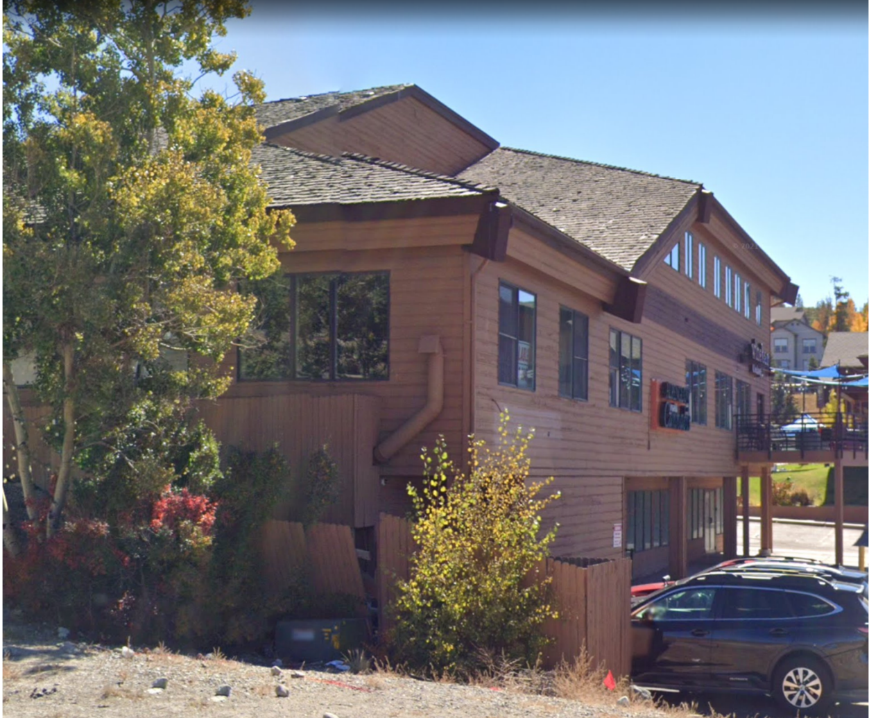
Side & Rear of the Building Where the Deck is Proposed
