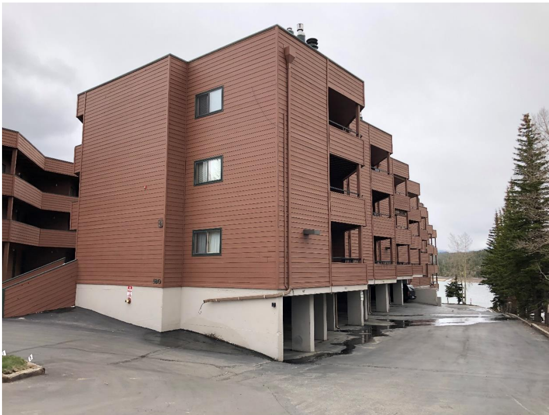
Tandem covered parking spaces at Marina Place Condos
