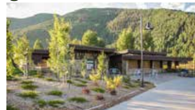
⑥ Concessions Building
