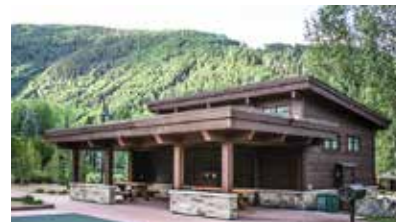
⑦ Lower Bench Restrooms
