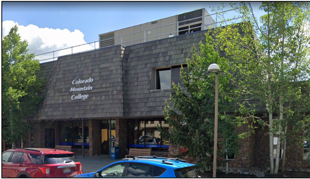
Figure 1. Roof Top Unit on Colorado Mountain College Building in Dillon’s Town Center
