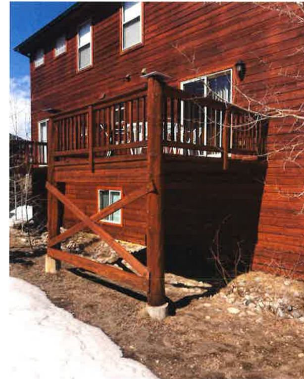
EXISTING DECK IN ANOTHER BUILDING SIMILAR CONSTRUCTION
