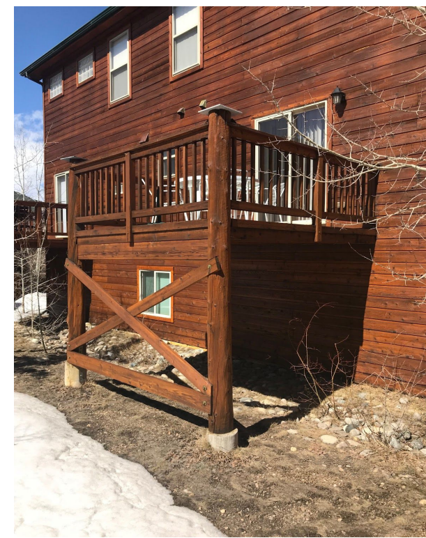
EXISTING DECK IN ANOTHER BUILDING SIMILAR CONSTRUCTION
