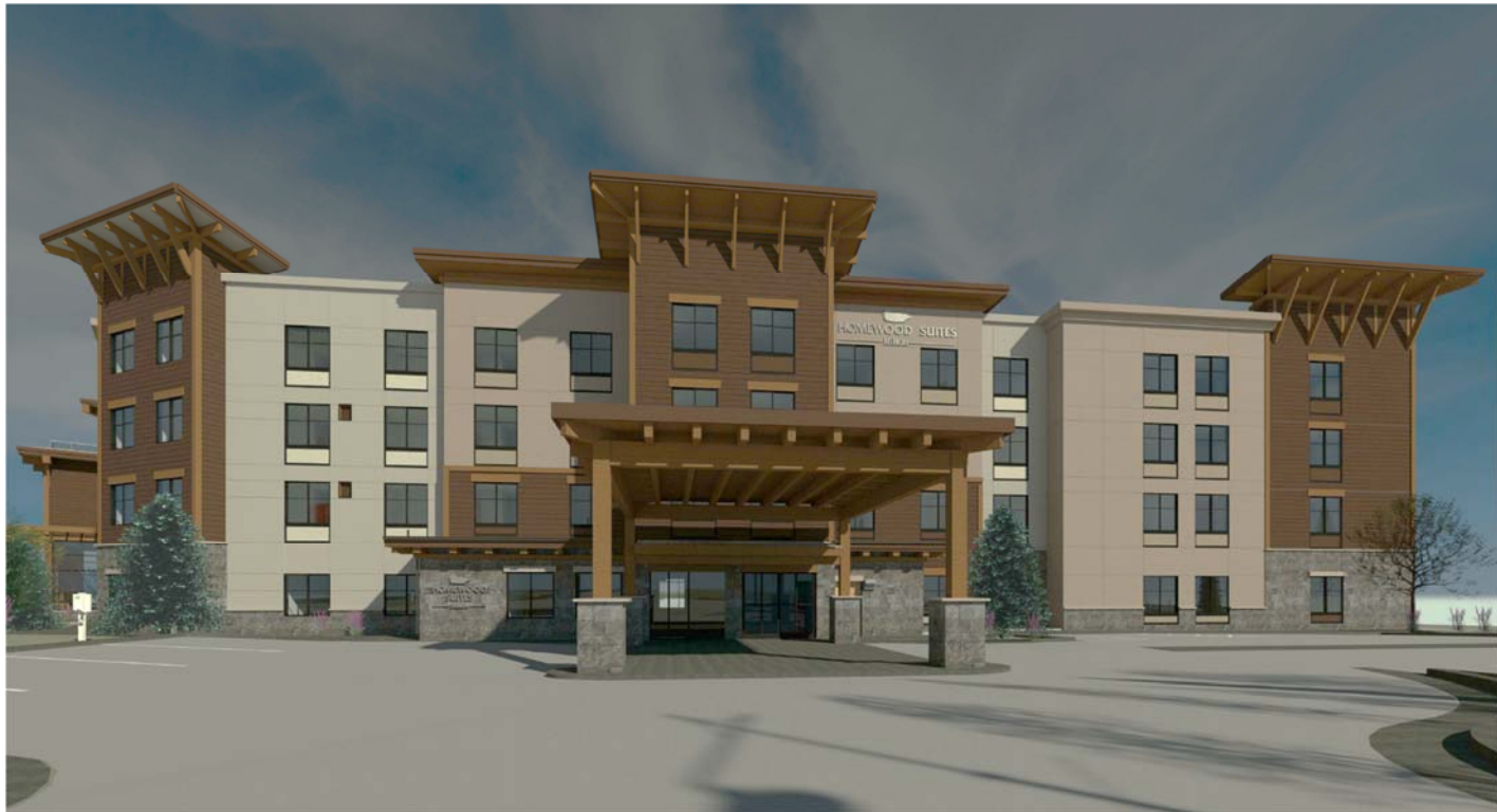
Figure 5. Beams, Roof Support Members, Roof and Façade Articulation, and Varying Siding Materials are Characteristic of the Architectural Design of the Building
