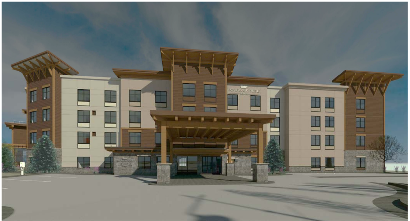
Figure 7. Beams, Roof Support Members, Roof and Façade Articulation, and Varying Siding Materials are Characteristic of the Architectural Design of the Building
