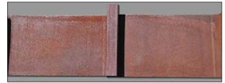
ROOFING FOR CABIN & LOWER UNIT 2 LOWER FLOOR:
