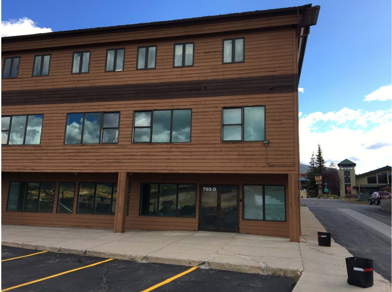
Rear of the Building Where the Deck is Proposed
