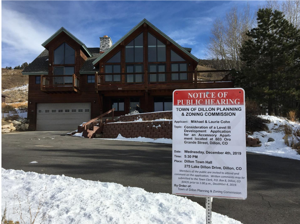
Site Posting November 25, 2019 - 603 Oro Grande Street, Dillon
