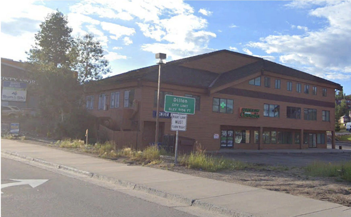
765 W. Anemone Trail, Dillon Factory Stores Building (© 2020 Google)
