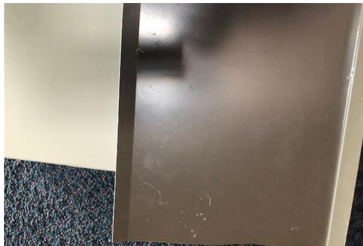
Natural Earthtone Colors: Beige building material and Brown trim and doors.
