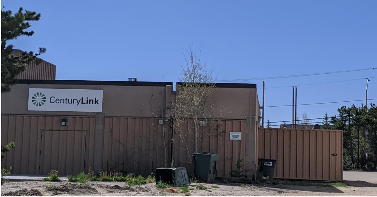
The existing CenturyLink building as seen from the 40' Right-of-way
