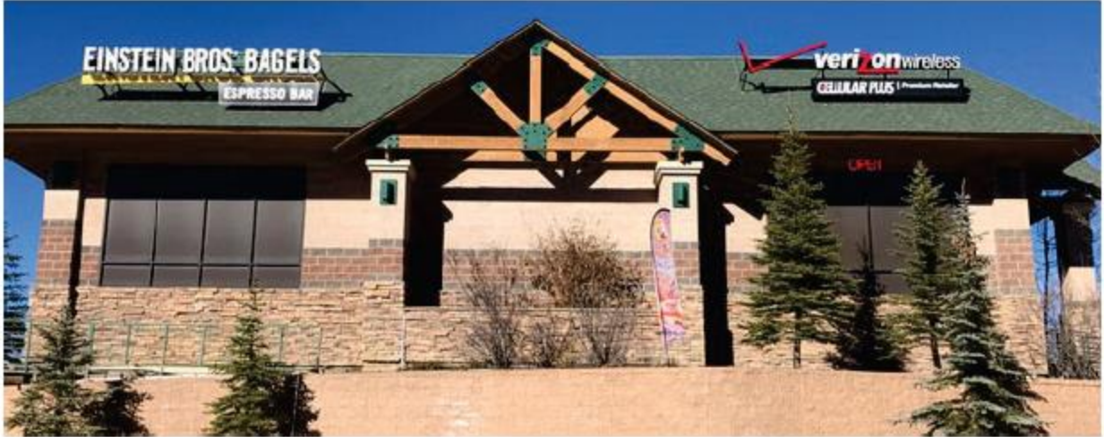
The existing tenant building signage on the southern side of the building at 35 Dillon Ridge Road
