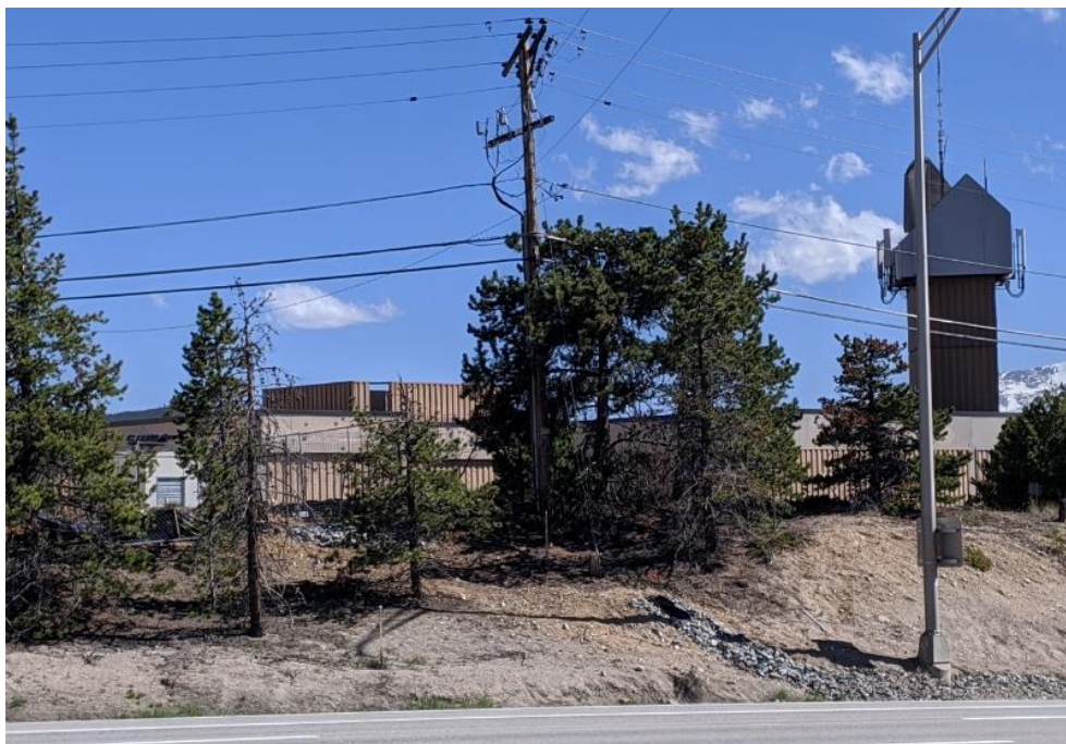
The existing CenturyLink building as seen from the US Highway 6
