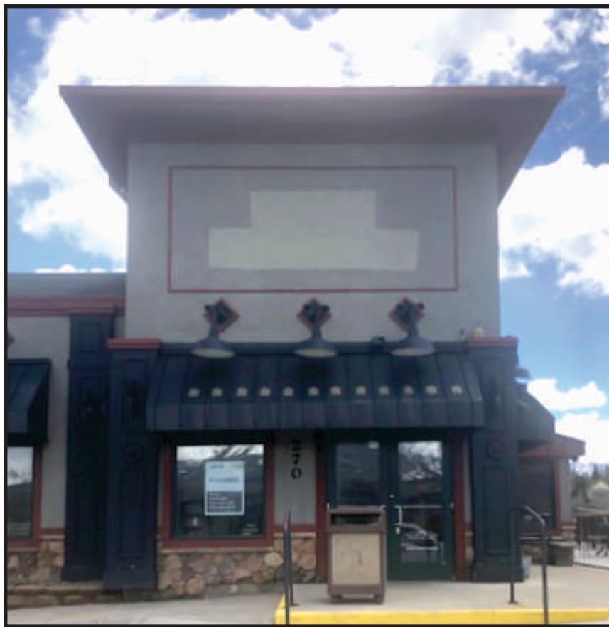
Existing Building West Elevation (BEFORE)
