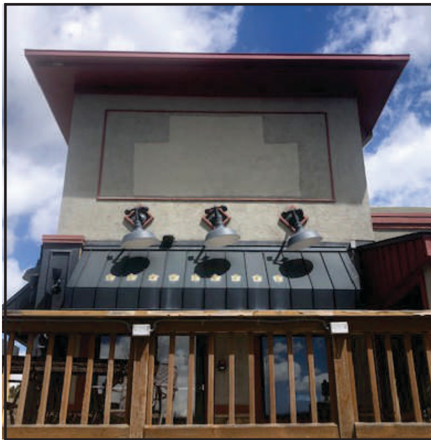
Existing Building South Elevation (BEFORE)
