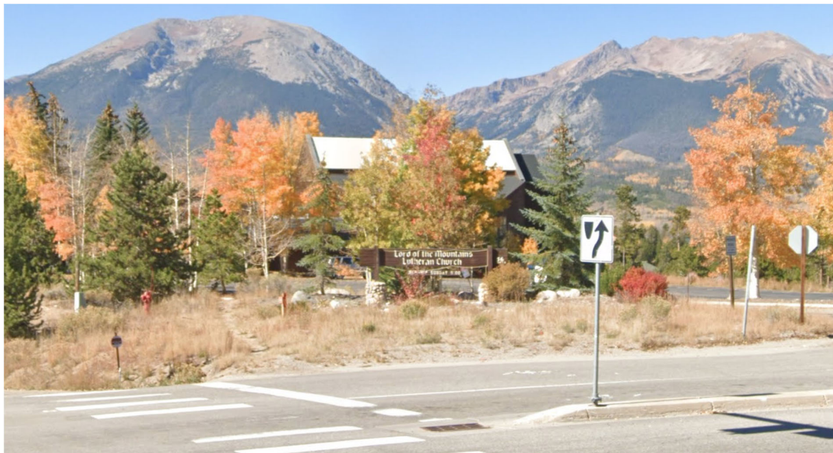
Figure 4. View of the Existing Location of the Lord of the Mountain Lutheran Church Freestanding Sign
