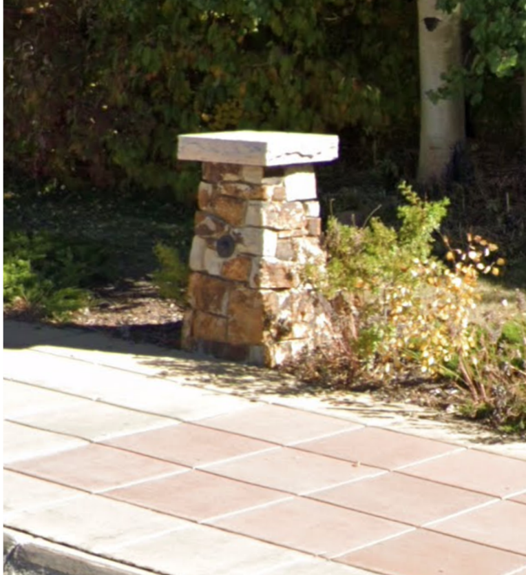
Figure 3. Stone Light Bollards on Lake Dillon Drive
