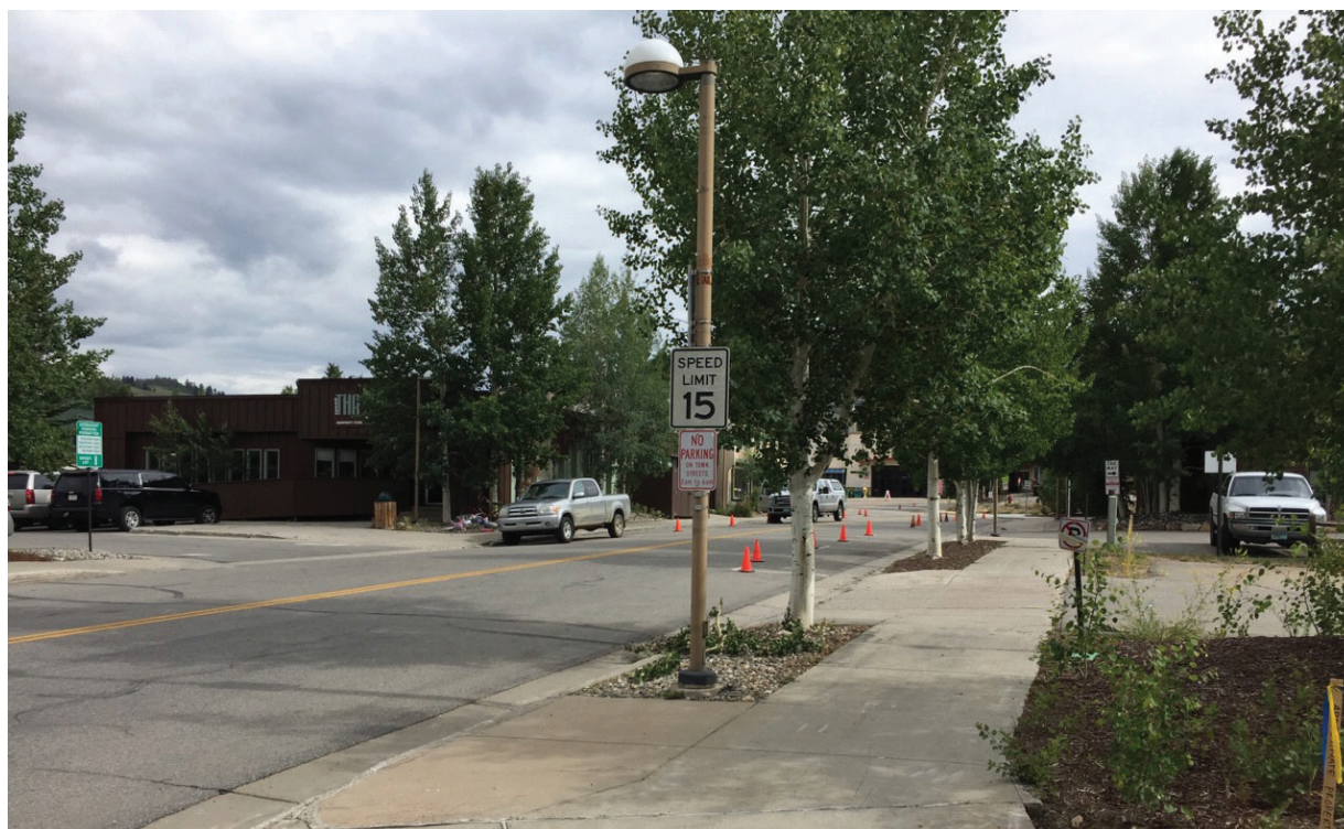
Fiedler Avenue at Colorado Mountain College
