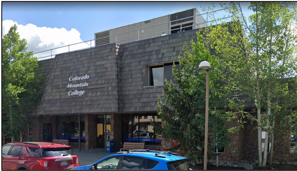
Figure 1. Roof Top Unit on Colorado Mountain College Building in Dillon’s Town Center.
