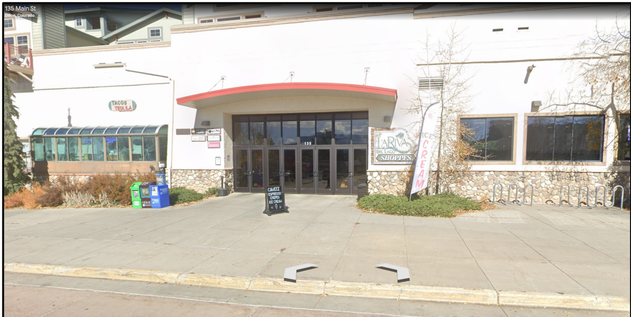
Figure 2. Existing Site Conditions as Viewed in Front of 135 Main Street (Source: Google)
