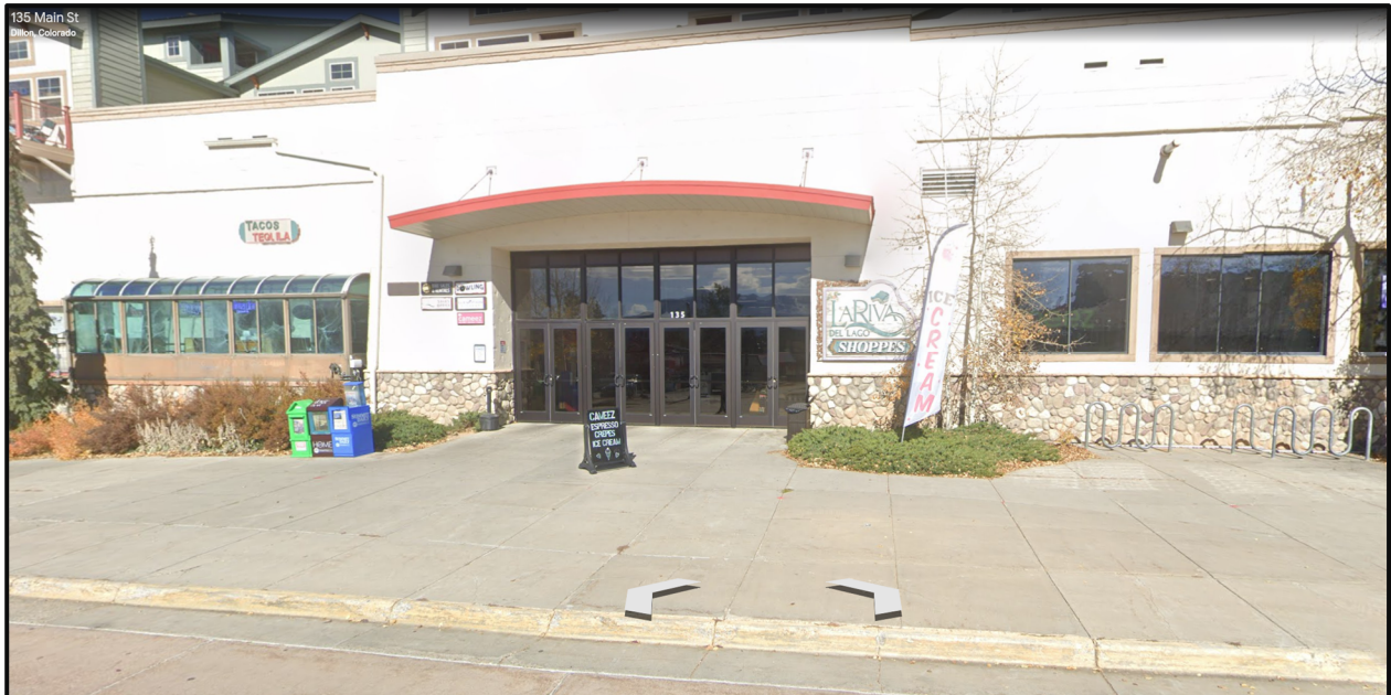
Figure 2. Existing Site Conditions as Viewed in Front of 135 Main Street (Source: Google)
