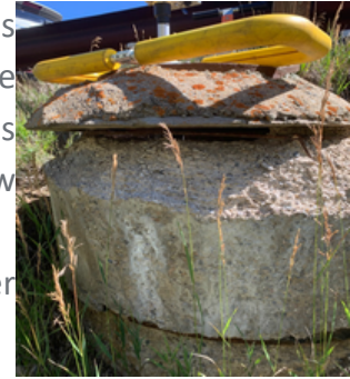
Manhole Repair in 2023
