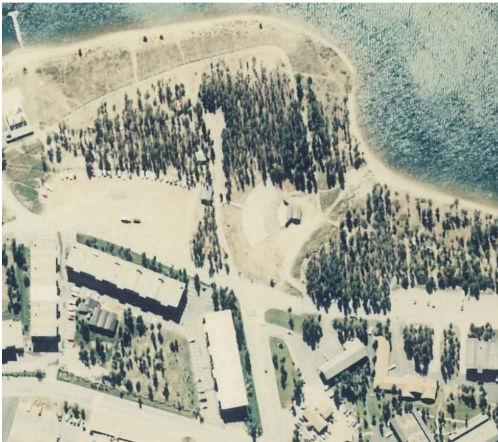
Dillon Amphitheater Aerial Photo Dated, September 22, 1991.
