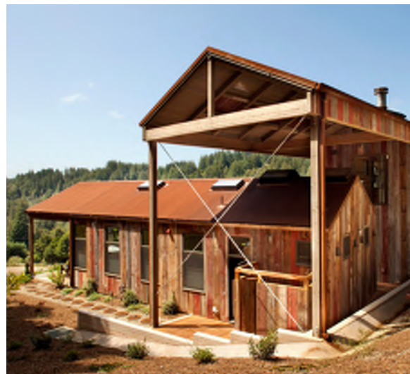
06. Aged and worn materials from the environment: stone, wood, and rusted steel
