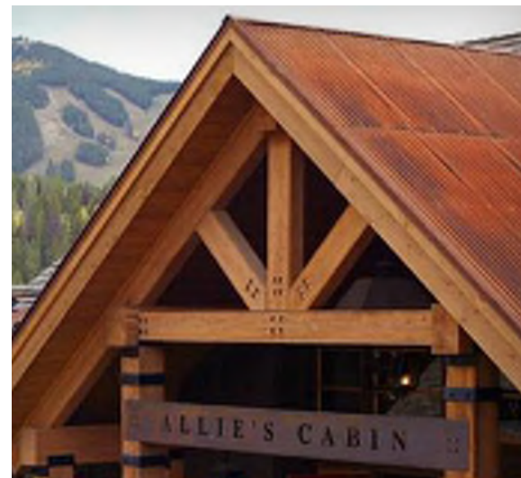
08. Heavy timber hardware connections: steel truss plates, column caps, connectors, tie rods
