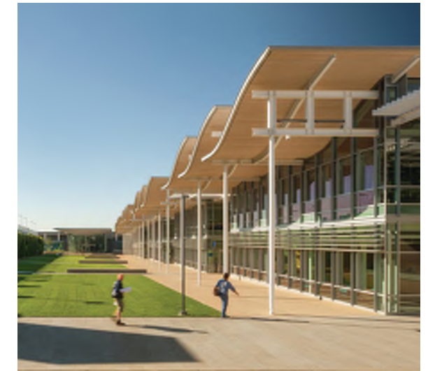
05. Floating roofs, and repetitive roof rhythms
