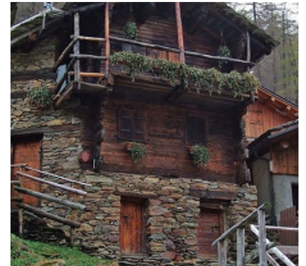
05. Substantial engagement/heaviness of structure with the ground
