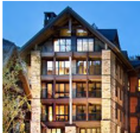
02. Pronounced post and beam Facade with Secondary Infill Windows
