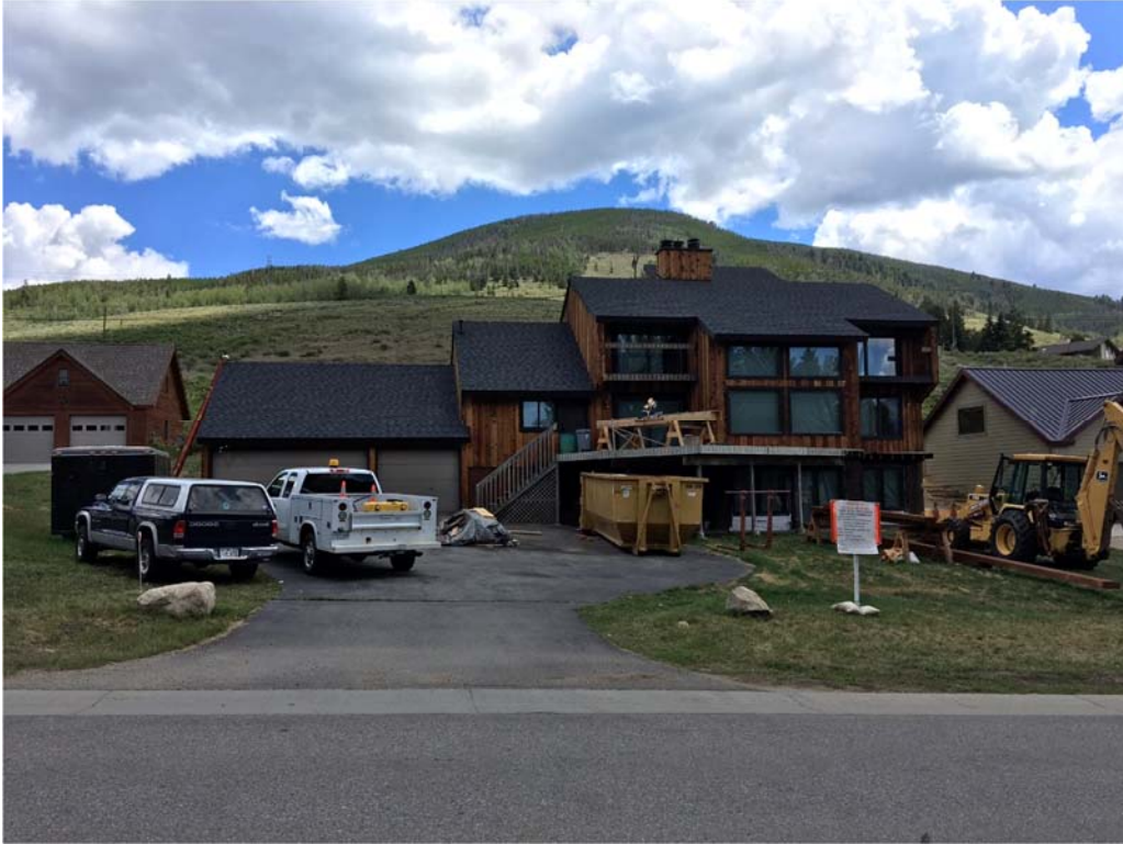
Existing Residence at 313 Tenderfoot Street.
