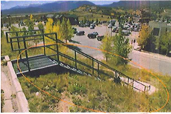
Dangerous slope for a business operating after dark
