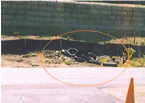
Rubble, weeds, open dumpster
